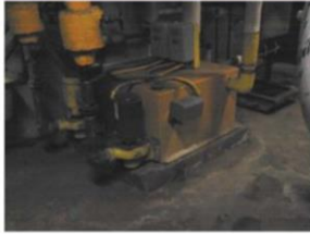
Insulated Condensate Receiver
