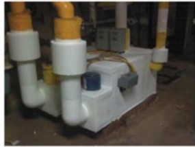
Insulated Condensate Receiver
